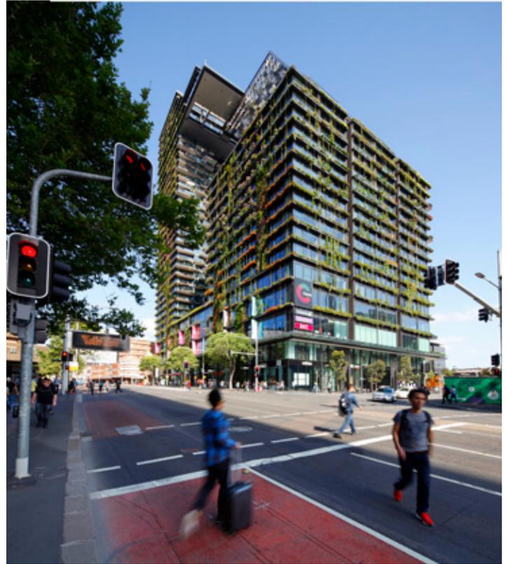
*The residential tower at One Central Park features a trigeneration system, water recycling plant and green walls irrigated with recycled water*
