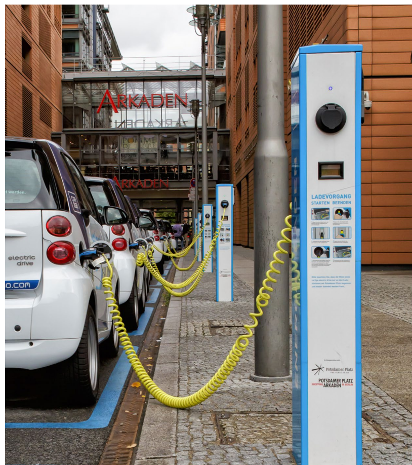
More present in the future’s cityscape: Chargers for electric cars
