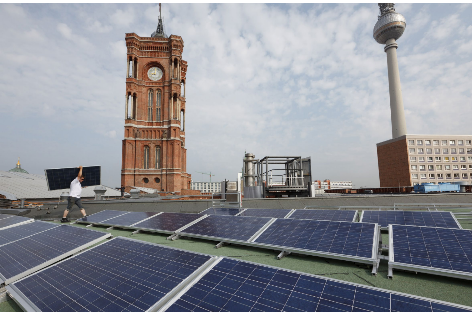
Assembly of the solar roof on the Red City Hall
